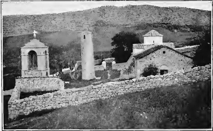
Fig. 1. THE CHURCH OF ST GEORGE AT KARDITZA, LOOKING TOWARDS THE END, WHICH IS MODERN
